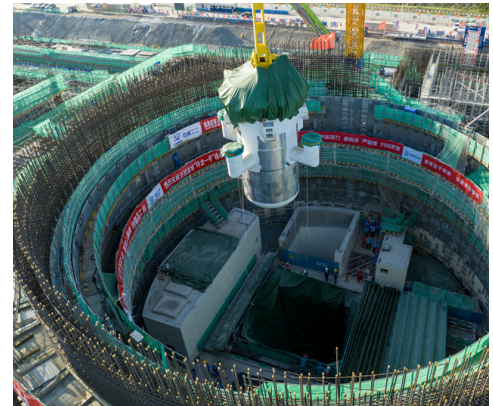
Fig. 1: The core module of the Linglong 1 SMR is lowered into place. Image courtesy of the China Atomic Energy Authority. Retrieved from https://www.caea.gov.cn/english/n6759361/n6759362/c10087720/content.html
